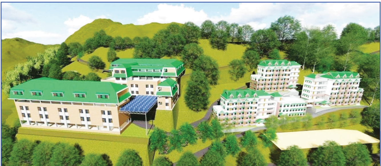
(3-D Image of HPNLU Under Construction Campus)
